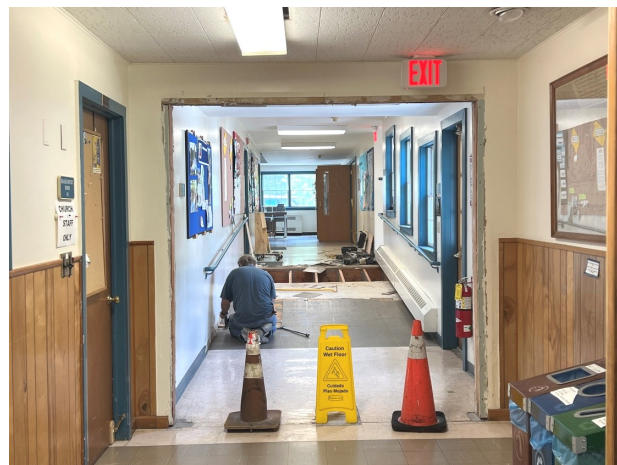
Office Hallway ramp Repair
